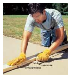
Cut in control joints
