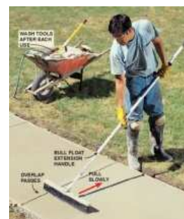
Broom the concrete
