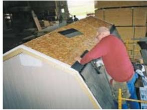
Now begin attaching shingles to the upper section. As shown above, fold shingle over the bottom section.
