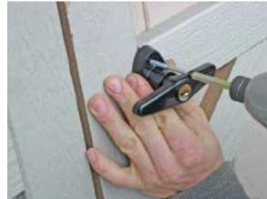
Position outside latch in alignment with drill points. Secure handle using two 2½" screws.
