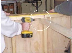
Locate the wall brace and secure to the center most 2X on one side wall. Note that the brace must be flush against the wall's vertical 2X and siding.
