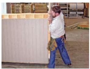
Note that the end wall section's base 2X will rest on the floor while the remaining 2X's will abut with the vertical 2X's on the side wall sections.
