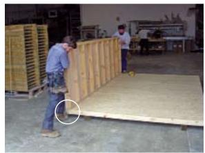
With the floor unit in its desired location, set the first side wall in place. The side wall's base 2X should set on top of the floor with it's siding overhanging the edge.
