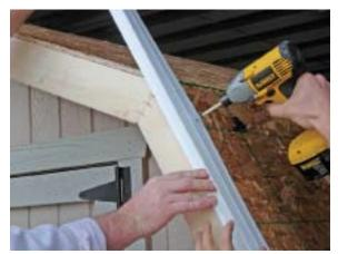
Continue to attach dripedge using 11/4" screws to the first bend.
