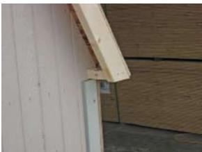
Repeat on the opposite end of rake. Then, attach the rake on the opposite end of structure.
