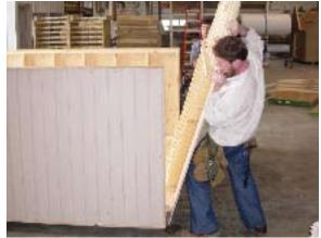
Locate the end wall section (without doors) and slide into place.
