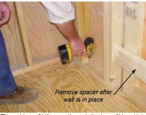
Then, drive a 2½" screw through the base 2X and into the floor at the opposite corner. Repeat steps #11 and #12. After wall is in place, remove spacer.
