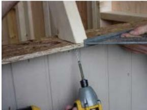
Use the angle square to ensure the cornered edge of truss and the edge of truss plate are flush. Then, drive a 2½" screw through the underside of truss plate and into the truss.
