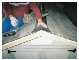
Beginning above the door, cut the ridge cap (as shown) and attach to roof.
