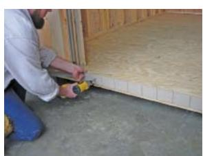
Locate the siding strip that fits below the door opening. Position as shown above and attach using 2½" screws every 8-12." Use a straight edge to ensure that the top of siding is flush with floor.
