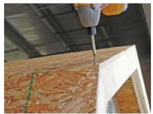
Secure ends of OSB to the rakes using 2½" screws.
