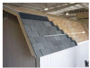
Install shingles across the entire lower section of roof.
