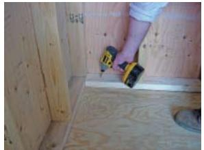
With the corners secure, now drive 2½" screws through the end wall's base 2X and into the floor every 16."
