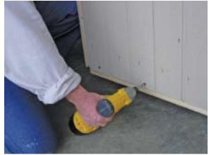
Secure the bottom of the end wall (w/o door) with 2½" screws every 12" (or every other board).
