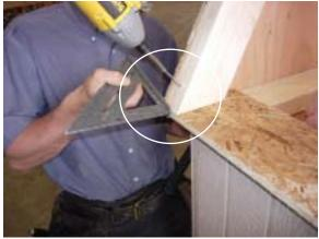
While holding the end wall in place, use an angle square to ensure that the end wall and side wall sections are flush. Then drive a 2½" screw through the 2X eave and into the side wall.
