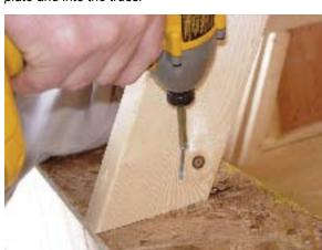
Toenail a third 2½" screw through truss and into plate below.
