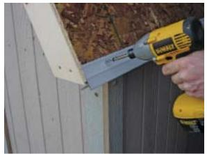
Install dripedge along sides of roof using 1½" screws every 1'.
