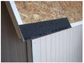
Align the top of starter shingles with the chalk line and attach.
