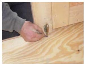
Hold the door in place (i.e., with door aligned to end wall and floor) and mark around the barrel bolt as shown.
