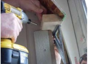
With all OSB panels in place, locate the rake block. Insert as shown above, using a angle square to ensure that it is level with the OSB and trim. Secure to wall using a 2½" screw. Repeat on opposite side.
