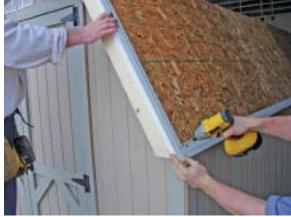
Then, install dripedge along the ends of structure using 11/4" screws, beginning at the front corner.
