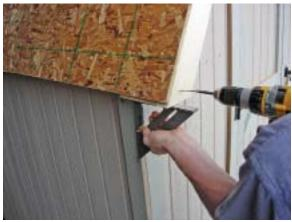
Use an angle square to square the rake with the rake block. Drive two (2)  $2\frac{1}{2}$ " screws through rake and into 2X framing.
