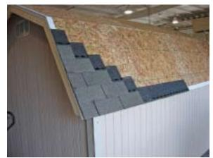
Add the second section of starter shingles. Then, stagger the next rows of shingles as shown.
