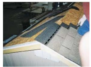
Continue attaching shingles to top roof section until reaching the ridge.
