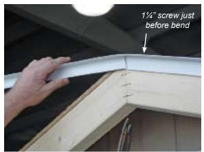
Secure the dripedge with a 11/4" screw just before the bend. Then, bend dripedge (along roof line) and attach along the remaining roof. Complete on the opposite end of structure.
