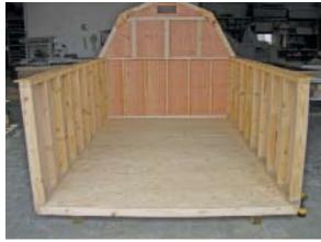
Locate the remaining end wall section with the door and set in place.
