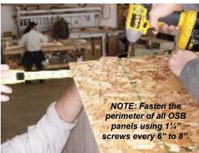
At the top, measure to a 6" overhang, adjust OSB as needed, and secure the OSB to end wall using a 11/4" screw. Repeat on the opposite end of structure. Then attach remaining top (then bottom) OSB panels.
