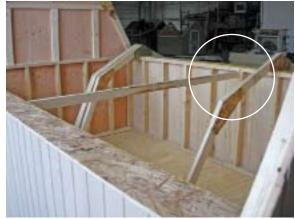
Push the side walls inward against the wall brace. Then, secure the wall brace to the opposite side wall in a similar manner.
