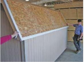
Snap a chalk line along the OSB consistent with the width of the starter strip. Consult the instructions provided with your shingle package.
