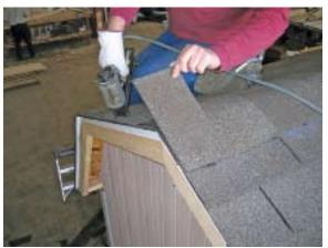
Once at the end of structure, finish the cap with a no adhesion strip.
