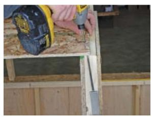
Secure the base of the OSB panel to truss using a 1½." At this point, attach only the bottom edge of OSB panel to each truss. Adjustments may be necessary.
