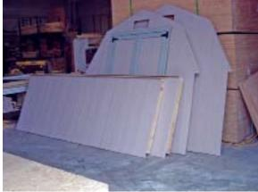
Place your materials skid in the exact location at which your building will be located. Remove the end and side wall sections from the materials and locate them close to your construction site.
