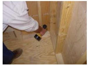
From the inside, drive a 2½" screws through the base 2X and into the floor at one corner.
