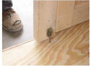
Drill hole using a 5/16" drill bit to accommodate the barrel bolt. Slide bolt into hole and verify (when closed) both doors are aligned with end wall.
