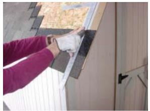
Once at the end of roof, use a metal square and <u>carefully</u> trim off excess shingles from the edge.
