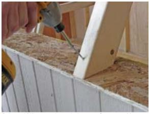
Drive a 2½" screw through the top of truss and into truss plate and 2X below.
