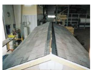
Complete the remainder of the top section. Then, install shingles to the opposite side of roof.
