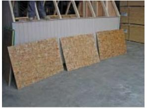
Beginning on one side of structure and consistent with layout diagram provided, situate the OSB roofing panels consistent with their designated locations.
