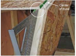
Raise the first OSB panel to position. Use an angle square to ensure that it's edge is flush with the corner of truss. Note that the edge of OSB panel must be centered along the truss' edge.
