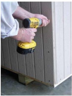
Next, secure the edges of the end wall with  $2\frac{1}{2}$ " screws every 12."
