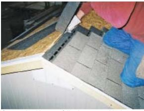
Once at the ridge, <u>carefully</u> trim excess shingle to expose ridge opening.
