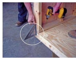
Use an angle square to ensure the end of wall is flush with the end of floor. Once flush and starting at one end, secure the wall to the floor using 2-2½" screws every 16."
