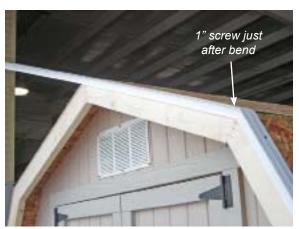
Bend the dripedge along the edge of roof, securing it to the roof with a 1½" screw just after the bend. Attach dripedge every 1.'
