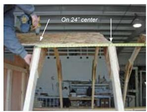
Using a tape measure, adjust the truss to a 24" center and secure the bottom of OSB.
