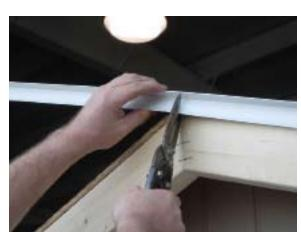
Once at the ridge of roof, again snip the dripedge to accommodate bend.
