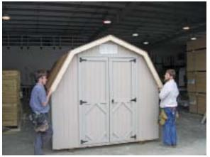
Raise the rake and set in place underneath the OSB sheeting and abutted against the 2X frame and rake block.
