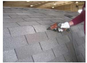
Once capped, staple shingles along the corners of roof line.
