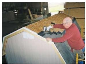
Continue attaching shingles to the top roof section, staggering in a shown.
