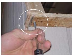
From below, drive a 2½" screw through the overhang and into the end wall's 2X eave. Then, repeat steps #11 and #12 on the opposite corner.
