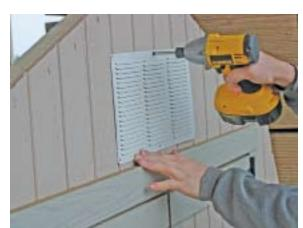
Align ridge vents around vent cutouts and secure using 1" screws.
