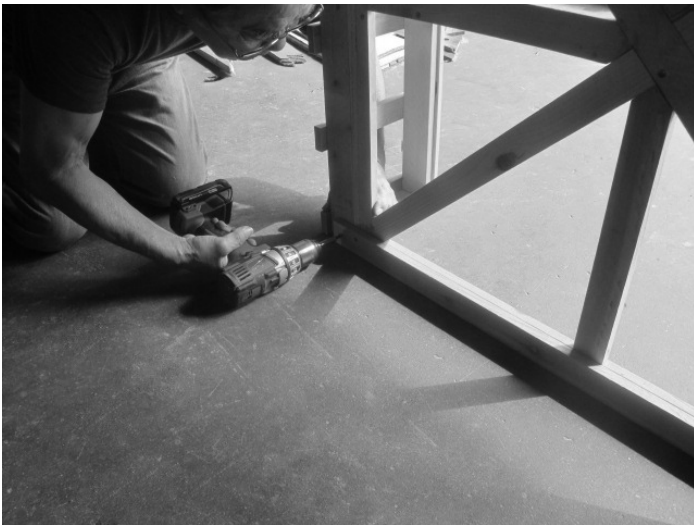
7. Fasten them with a screw at the bottom.
