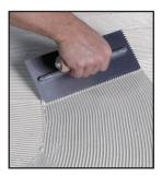
backing; remove adhesive and reapply. *After Installation* – Restrict foot traffic and moving of heavy objects for 24 to 48 hours to allow adhesive to cure properly. Premature traffic can cause installation failure.
