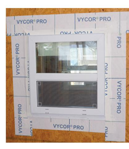
A properly integrated flashing tape that adheres and seals aggressively to the substrate will create the most effective barrier against water and air migration while acting as a drainage plane to shed water down the exterior of the building envelope.
