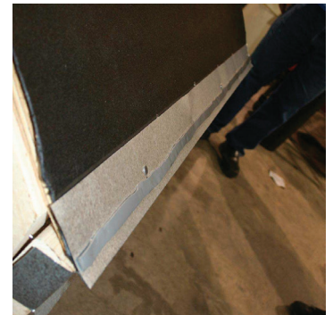
Inspect the tape to ensure there are no gaps or breaks
