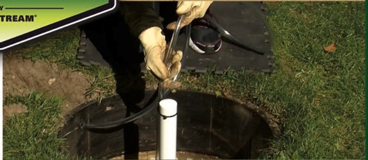
Use tubing to lower diffuser into tank liquid
