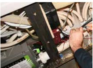
**STEP 3** - Uncouple on/off switch to MP3 allowing you to remove the panel away from the spa and gain access to the pump.
