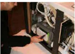
**STEP 4** - Unscrew face plate of control box using screwdriver
