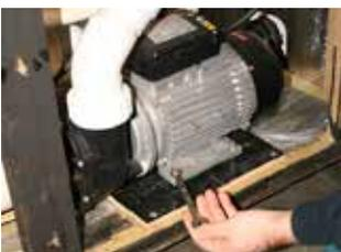
**STEP 8** - Remove all 4 nuts from pump base using a 51/8”(13mm) wrench
