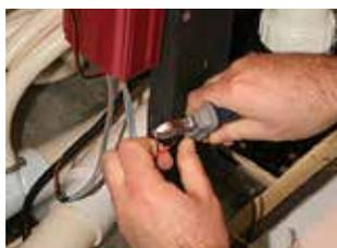
**STEP 6** - Remove insulation from speaker wires and join using 5A connection block (Red to Red and Black/Red to Black/Red)
