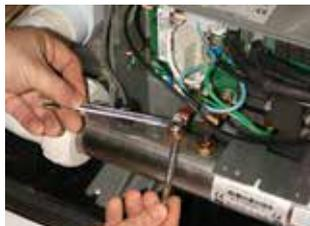
**STEP 6** - Unscrew heater nuts using 3/8 inch+9 wrench underneath copper jumper and hold in place while unscrewing top nuts using a 6 mm spanner
