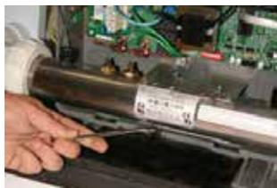
**STEP 7** - Unscrew both locking nuts on heater from brackets using 6 mm spanner
