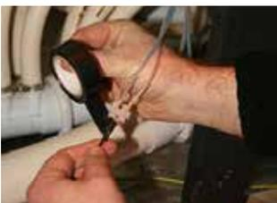
**STEP 10** - Insulate tape connector and wire
