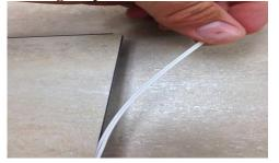
Overlapping the SimpleFit® Locking Strip over the previously installed plank/tile
