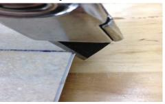
Locking long tongue into groove and slide at a low angle until first inch of the SimpleFit® Locking Strip touches the short groove edge of previously installed plank/tile
