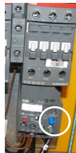
C. Once motor has cooled, press-in on BLUE button
