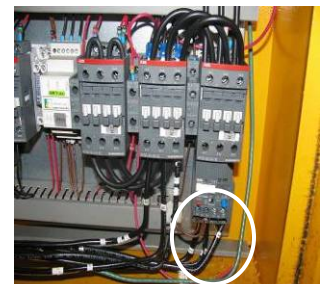
B. Locate BLUE reset button on relay attached to K1 contactor.
