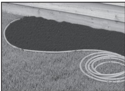
**1.** Define the shape and location where you wish to install the StoneWall Border (e.g. a garden hose works well). Clear the edge area of grass, rocks, roots and other debris, and smooth the ground as much as possible.
