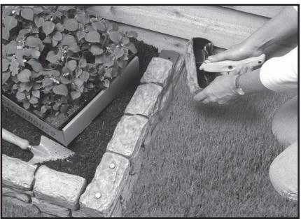
**6.** At the end of a freestanding wall, you may cut off half of the Bridge Piece, which is easily done with a box knife or hand saw (*the inside of the Bridge Piece is already indented to facilitate cutting*), and install it on the Base Piece with the solid end positioned on the outside.
