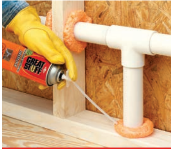
Seal pipe penetrations
