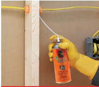
Seal Electrical Through Wall Studs
