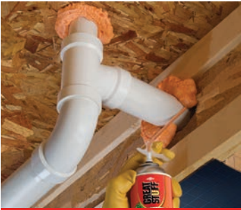
Seal pipe penetrations
