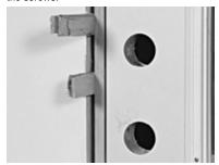
Shim behind the latch-side jamb approximately 8" from the top and bottom of the frame. Install shims until there is an even 1/8" gap between the jamb and the edge of the door slab along the wholee length of the door. Shim behind the latch-side jamb just above and below the deadbolt hole, maintaining the 1/8" gap. Pull the weatherstripping away from the jamb and screw 3" installation screws through the jamb and shims and into the stud.
