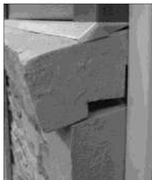
Window and Door Trim under the Ledger
