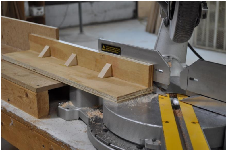
Construct jig to match bar rail installation
