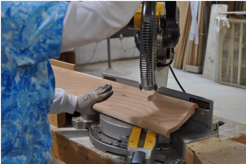
With bar rail in position cut at desired angle with saw vertical
