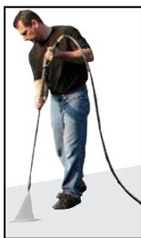
**OPTION#1 - PRESSURE WASH:** For easiest and most effective cleaning results, use a minimum 1800 psi pressure washer to thoroughly remove embedded dirt and all cleaner and etching residues. Hold the tip 6 inches from the surface and use a **SLOW sweeping motion** across the surface. When pressure washing is complete. Let the surface dry 1-2 hours before application (longer in cool, damp or humid conditions).
