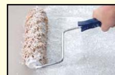
2) Apply RollerRock over the stenciled surface and allow it to cure for 24 hours.
