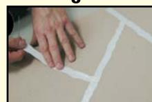
1) Lay DAICH flagstone tape onto primed surface in desired pattern.
