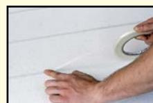
1) Lay DAICH grout tape onto primed surface in desired pattern.
