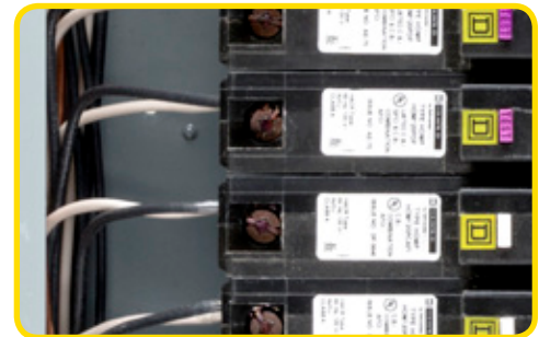
▲ Plug-on Neutral connection
