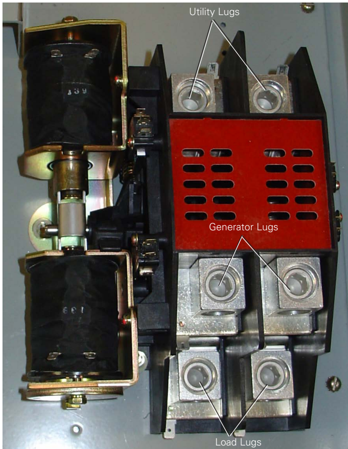
Figure 15. Cable Connection Locations (200 A Shown) Typical.
