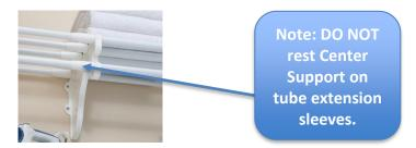
14. Attach Center Support using anchors and screws (see steps 4-5 on page 1).
