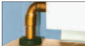
**Fast/Flex connectors** can be hand formed around obstructions, go through tight spots and make up for any misalignment between baseboard and piping. Here, one Fast/Flex replaces three elbows and three lengths of tubing, eliminating much measuring and fitting. (See Pub. No. EC-FF-10 for additional data.)
