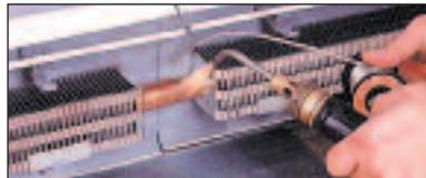
**Vented return bend.** Special 180° bend aligns return line perfectly with half-moon cutouts in support brackets. A ½" threaded tapping permits easy installation of air vent, can also serve as a drain
