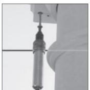
Apply construction adhesive\* to top of cap, press against structure, and screw or nail into place.
