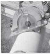
**2.** Use an abrasive saw (masonry or carbide tip blade). Fine trim top and bottom with rasp to assure flat surface contact.
