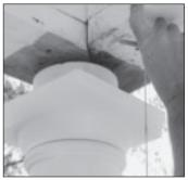
3. Slip base over top of column shaft and allow to slide to base of shaft. Slip cap over shaft and allow to rest on neck mold. Some sanding may be required.
