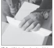
**10.** Pre-drill holes through neck mold into column. Screw neck mold in place or pre-drill and use finish nails.
