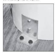
**6.** Mark and drill holes in floor and column shaft for corner/ angle brackets (not included). (HB&G column installation kit available #17040)
