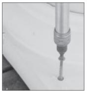
**8.** Apply construction adhesive\* to bottom of base and nail or screw to floor.
