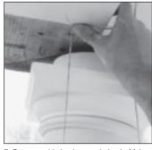
**5.** Put assembly in place and plumb. Make sure load is centered over column shaft and evenly distributed around the bearing surface.
