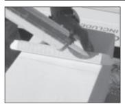
**9.** Mark location for supplied neck molding. Measure and cut neck molding to a 45° angle. Apply construction adhesive\* and put neck mold in place.
