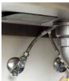
both below the sink and in the basement. Once you find the valves, open and close them to make sure they are functioning properly. It is important to check these valves often, as they may become “frozen” from lack of use. Usually a wrench applied to the control handle will free up the valve, turning clockwise to start to close the valve since it is probably in the open position. However, do this carefully to avoid breaking off the control handle.
