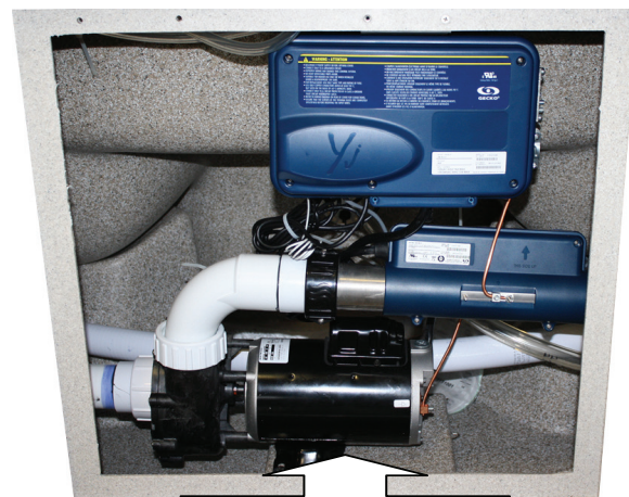
230 Volt Equipment Compartment
