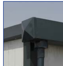
Rear Water Gutter System
