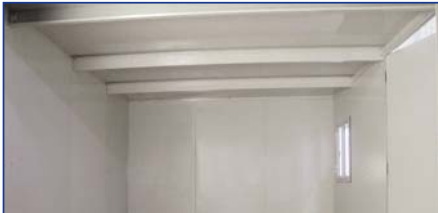
Building reinforced with metal columns and beams
