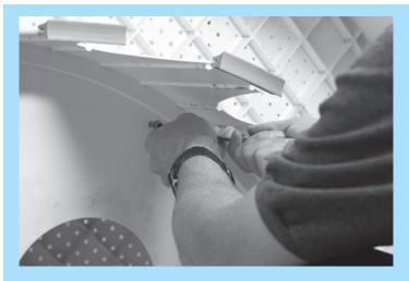
Once the 9 holes are lined up secure the base step to the step assembly until all 9 screws are in place along with the stainless steel washers. Be sure to hand tighten only using the screw driver that comes with the step.
