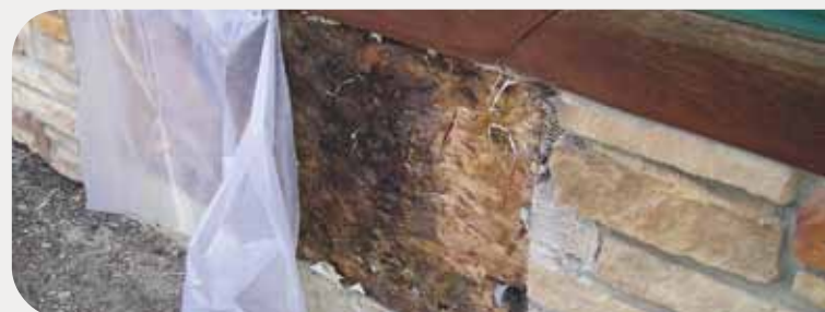
Once moisture gets in, it has nowhere to go, creating the perfect environment for mold growth and eventual structural failure.
