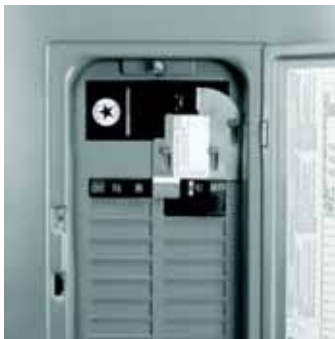
Cutaway Showing Installed Generator Interlock Kit
