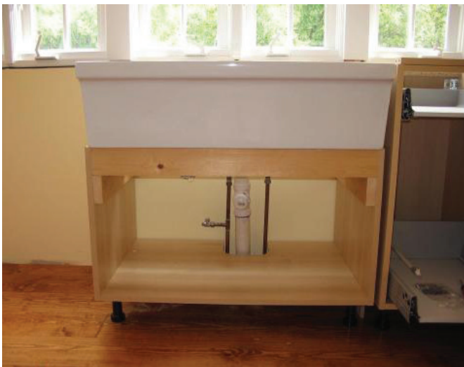
[Above]: Cabinet and sink in place.
