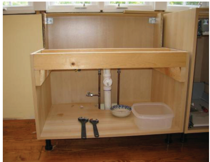
[Above]: The cabinet is now fully installed, and ready for the sink to be set in.
