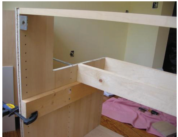
[Above]: Details of the support structure from the back.
