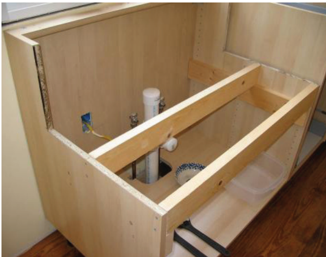
[Above]: The cabinet is lifted up over the plumbing, and set in place
