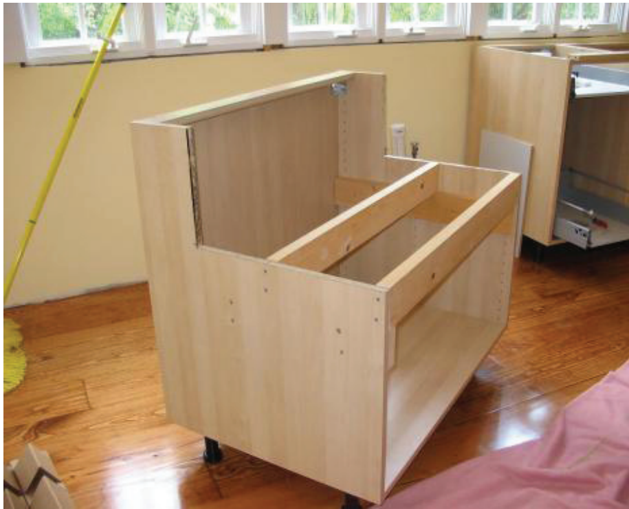
[Left]: The back of the cabinet is nailed on, and now the modification of the cabinet is complete.
