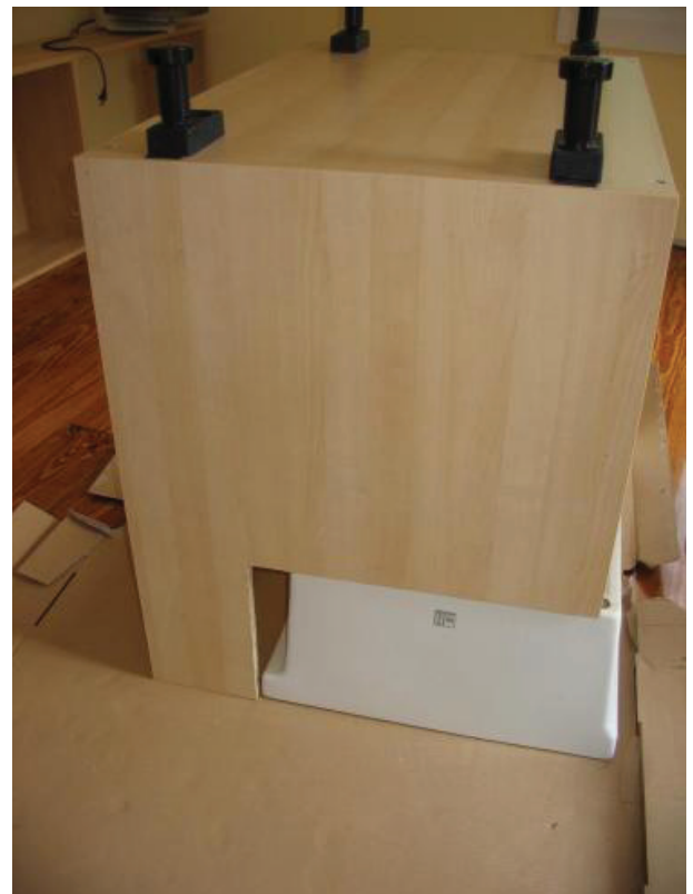
[Right]: Then, to check the fit, turn the cabinet upside down over the sink. Why did we do it this way? Because right now, there is nothing to support the sink. The sink tapers and is too narrow at the bottom to sit on the cabinet sides.
