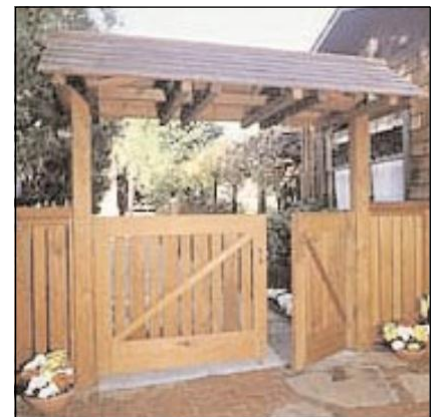
Rooftop-style canopy over a Craftsman fence shelters the entrance beneath it. Shingles on the canopy echo the design of the home. Posts are 6x6's and support the 4x4's of the canopy.
