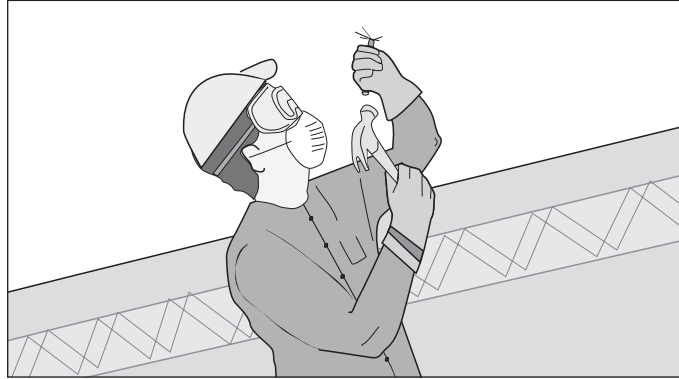
Fig.5. Make an initial hole.
