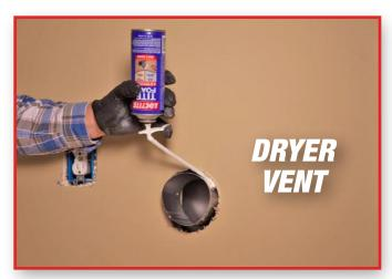
Block out pests and eliminate air infilitration by insulating the gap between the dryer vent and dry wall.
