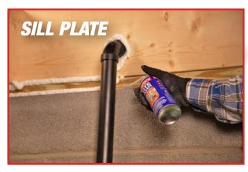
Use foam to insulate the gap between the wood and concrete to prevent heat loss.
