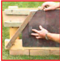
Angles for Roof/Hanging Tiles
