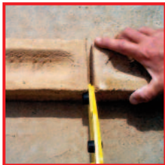
Gauge 10mm Standard Brick Joints
