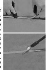
wrapper will liquify immediately, continue to move the flame back & forth, side to side, in a slow even manner, heating about one foot at a time. The stix will start to liquify immediately but you should continue heating for about 1 - 2 minutes. The type of torch, along with wind, temperature conditions, and thickness of stix will affect melting time. Traffic Ready in approximately 20 minutes.
