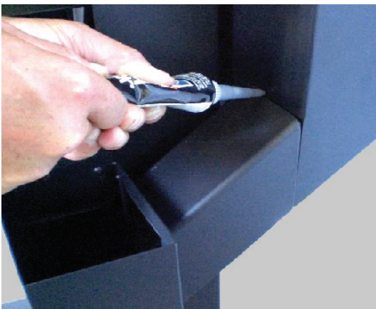
Apply silicone around all four edges
