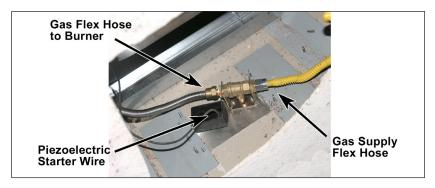
Place the fire pit back down on its pedestal. Attach the gas flex hose to the burner.
