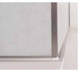
QUADEC square-shaped profile and corners used to finish the tile edges on the wall. QUADEC-FS double-rail edging profile used to frame the mosaic insert in the wall. DILEX-AHK cove-shaped profile and corners used to create a smooth transition between the floor and wall.
