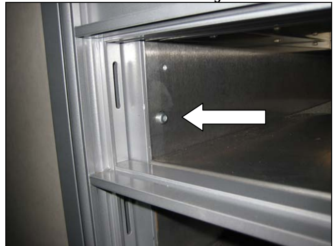
Illustration 3 - Location of Mounting Hardware Hole
