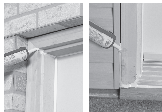
Figures 31 and 32 : Caulk the jambs and the exterior trim.
