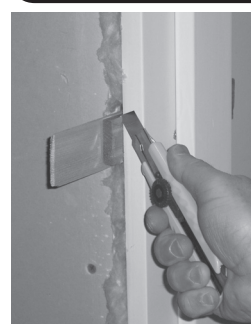
Figure 28 : Insulate between the jambs and the wall studs all around the door.
