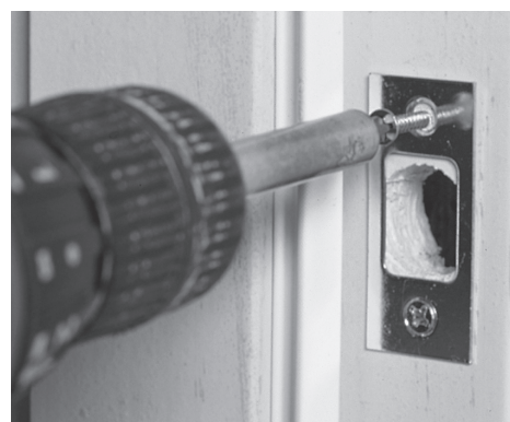
Figure 26 : Screws fasten the latch plate to the door slab.
