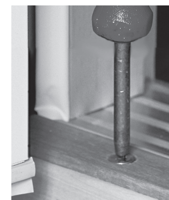
Figure 33 : Raise or lower the sill by adjusting the sill screws. Some sills may have covers over the adjusting screws. These covers must be removed prior to making any adjustments.
