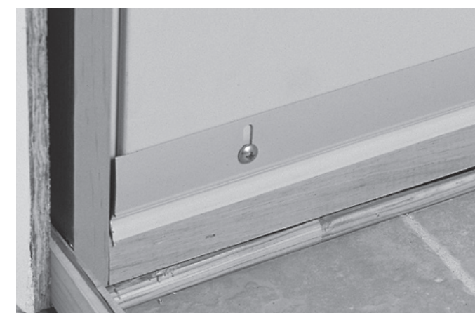
Figure 34 : U-channel sweeps are adjusted to form a tight seal with the sill.
