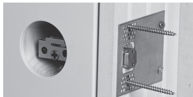
Figure 27 : Screws should connect the dead bolt plate to the stud.
