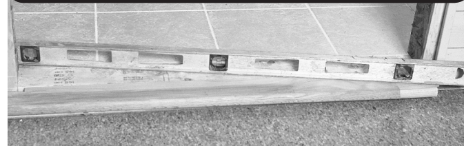
Figure 1 : A clean, level, solid sub-floor area is essential for successful installation.
