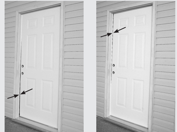
Figures 9 and 10 : The weatherstripping on these doors is not evenly compressed.
