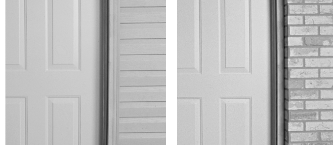
Figures 7 and 8 : The exterior trim (brickmould) rests up against exterior sheathing or slides into the opening of exterior brick.
