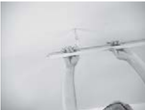
Install first main beam
