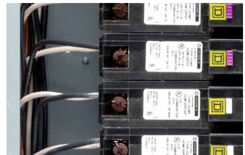
▲ Plug-on Neutral connection
