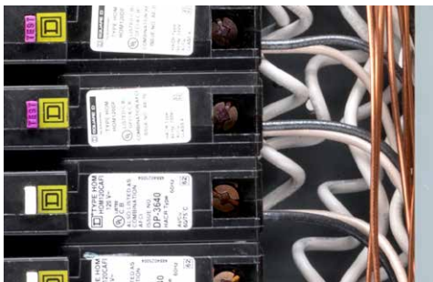
▲ Pigtail Neutral connection
