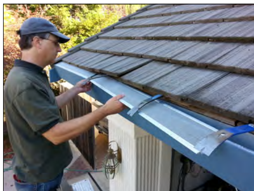
Flat bars used to lift up tile.
