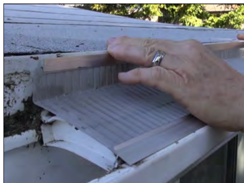
Bending mesh to fit small gutters.
