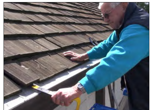
Using flat bars to lift up wood shake.
