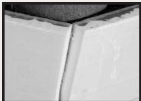
Imperfect edges are easily hidden under grade or by the siding or J-channel. For perfect edges use a circular saw with a masonry blade.
