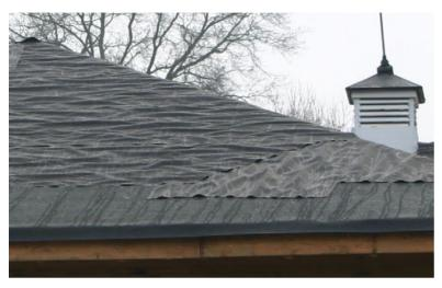
Conventional organic felts can absorb moisture, causing severe buckling and wrinkling—and a terrible-looking roof
