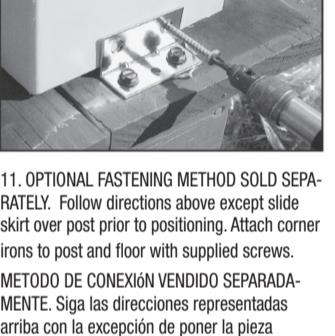
11. OPTIONAL FASTENING METHOD SOLD SEPARATELY. Follow directions above except slide skirt over post prior to positioning. Attach corner irons to post and floor with supplied screws.
