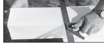
3. If using handrail, check local building codes for minimum rail height. Decide how much is to be trimmed from each end of PermaPost. Top and bottom mounting plates combined are 3/32" thick. Mark post 1/16" shorter than total opening.
