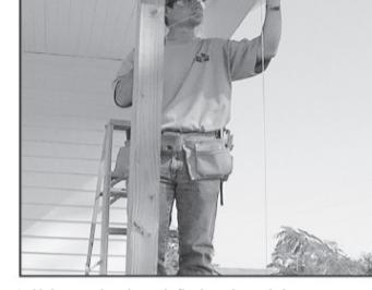
5. Fasten one plate, edges down, to the beam above.
