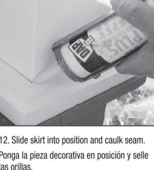
12. Slide skirt into position and caulk seam.
