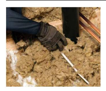
Gaps and voids in the attic can account for up to 30% of the heat loss. Areas around pipes, wiring and attic vents are often neglected and can account for the majority of those gaps and voids. ROXUL ROCKFILL™ loose fill, top up attic insulation makes it easy because unlike other attic insulation, there is no blowing machine required, and installation can be done by hand.
