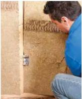
ROXUL COMFORTBATT® higher density batts make it simple for precise cutting to ensure a fit without gaps and voids.
