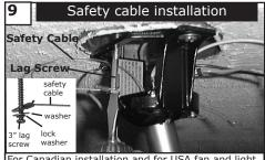
For Canadian installation and for USA fan and light kit combinations over 35 lbs, in both flush and downrod modes the safety cable must be installed into the house structure beams using 3" lag screws, washers and lock washers provided. Make sure that when the safety cable is fully extended the lead wires are longer than the cable and no stress is placed on the lead wires. **Note**:If Installing The Secondary Support Safety Cable in the U.S., Do Not Remove Knockouts In The Outlet Box.
