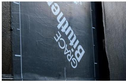
Fully Adhered — Forms integral bond to substrate Keeps basement dry and comfortable
