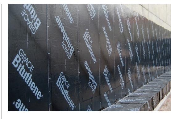
Grace<sup>®</sup> Bituthene<sup>®</sup> fully-adhered waterproofing membrane is applied to the outside of basement walls. Its cross-laminated film ensures a waterproof seal. Protect your project with Grace Bituthene<sup>®</sup> waterproofing membrane for a durable and watertight below-grade solution.
