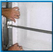
Step 5: Insert the insulation sheet between the horizontal rails.
