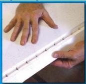
Step 4: Insert the excess insulation behind the vertical rails
