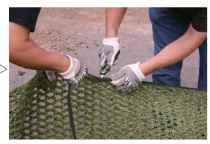
Cutting the selvedge will prevent from wrinkling up. It will be much easier to pull and stretch out to get best installation.
