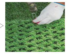
Nail down one side first, this will make installation lot easy (after one side installed, be sure to pull and nail the other side for tight installation).
