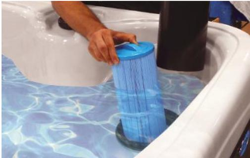
Unscrew the cartridge and remove it.
