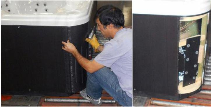
Then, unscrew and remove the front door panel.
